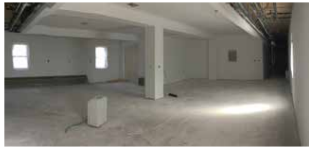
The "unfinished space" (now partly finished) seen from outside door. Opening of "tunnel" to our basement visible back right.
